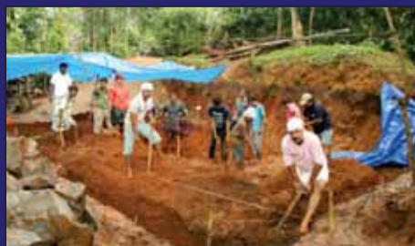
Jijo Kuriappan (at front) leading the basement-laying work
